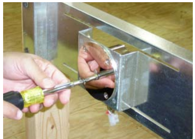
SolidDrive SD1 drywall installation during new construction View from behind
